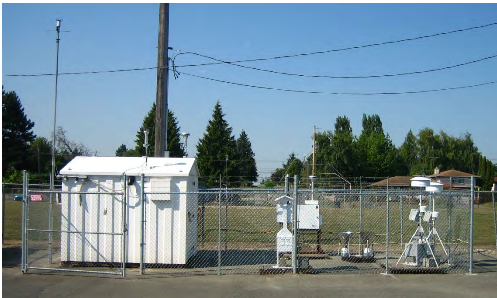
Figure A-10. Tacoma South L monitoring site photo
